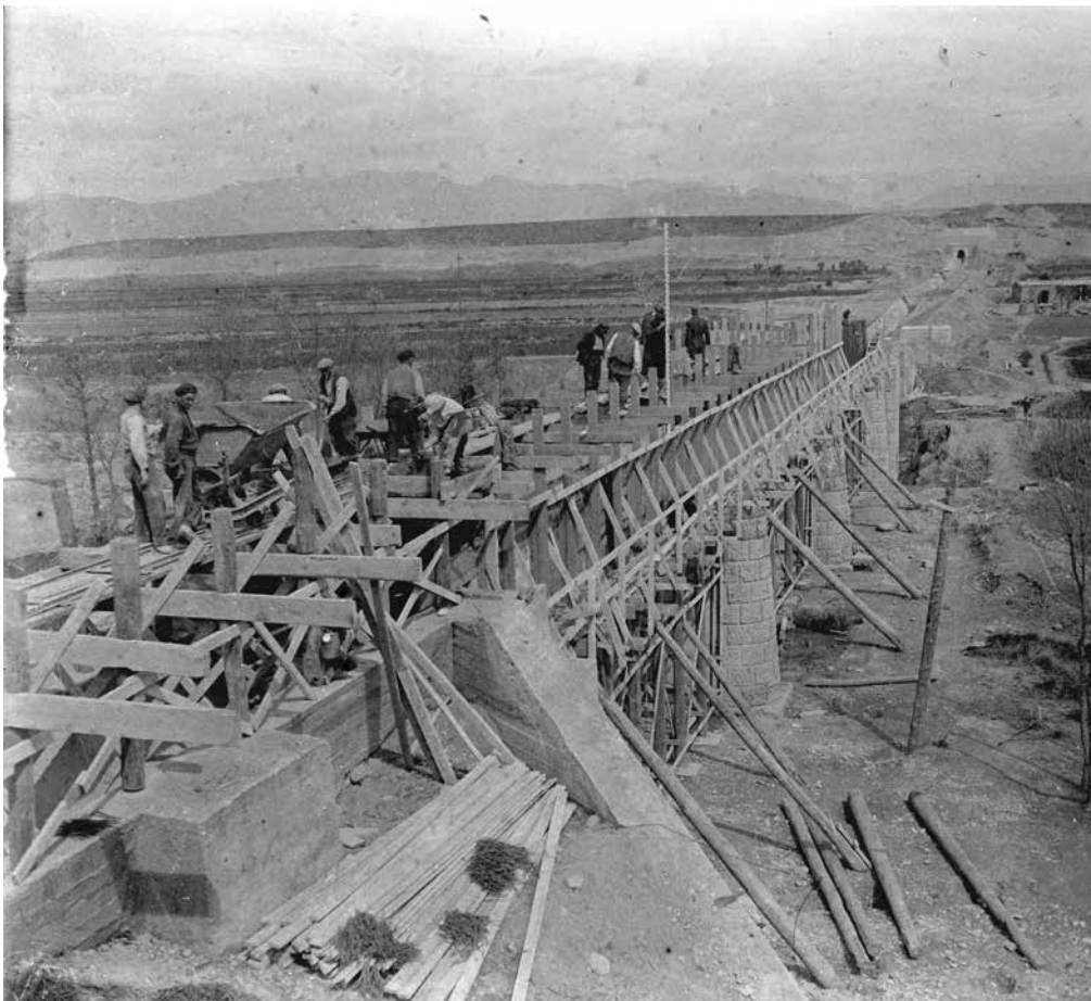
Urgell canal construction works at the end of the nineteenth century
